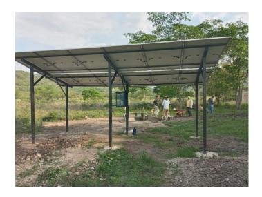
In addition, a superficial water pump with 8 solar panels of 400 watts was installed with a hydropneumatics tank with a capacity of 120 gallons to keep the pressure in the system due to the flat geography of the community. The community will have running water for about 10 hours a day, every day from 7: 00 am until 5:00 pm and the system will also have the option of using the grid system if necessary.
